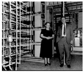
Crown Point Telephone Corporation central office with S.C. X-Y switch c. 1950s
